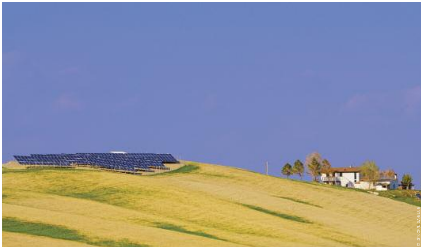
image SOLAR ENERGY FOR A COUNTRYHOUSE IN TUSCANY, ITALY.
